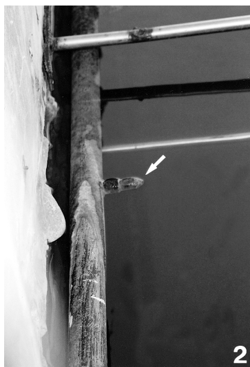
Photo 7-2 : Water massage system. Arrow indicates a nozzle expelling hot spring water into pool for massage.
