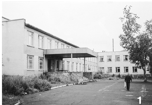
Photo 1-1 : Main building of the sanatorium.
