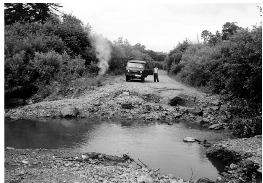
Photo 7 The scene of collapsed bridge on the road of the Sikhote-Alin crossing road.
