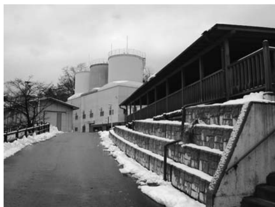
Photo 3 Kusatsu Neutralization Plant (Shinaki Dam Water Quality Control Office, December 23, 2007).
