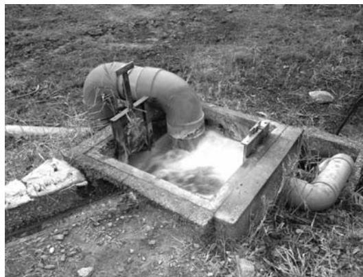
Fig. 9 Drilling well of Tezuna hot spring source. 3,000 l /min.
